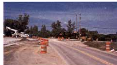
The Little Blue Parkway Intersection with 39 th Street under construction (looking north)
