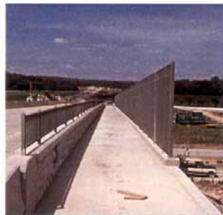
The bike lane enhancement to the Little Blue Parkway bridge over I-70 are a good example of quality community design (under construction)
