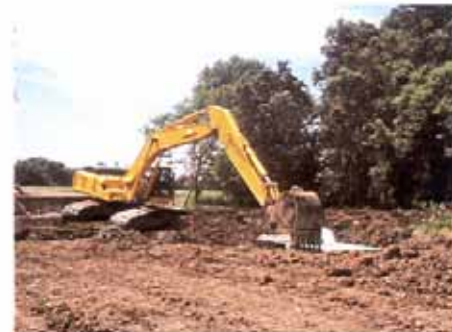
Tapawingo Sewer Interceptor under construction
