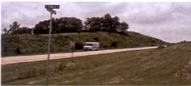
24 Highway just west of Powell Road; the future terminus of the Little Blue Parkway
