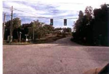
The 40 Highway and Little Blue Parkway Intersection under construction; the Southern terminus of the Little Blue Parkway.
