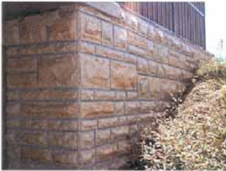
Enhanced poured limestone facade given to the Little Blue Parkway Bridges over the Little Blue Trace and Interstate 70
